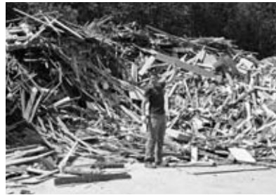
documentation still Rohbau 2007
